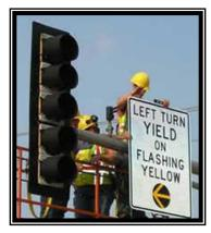
ed several benefits from placement of the flashing yellow arrow. The new signal allowed more traffic to move through an intersection, provided additional traffic management flexibility, provided motorists with a clear distinction of yielding to oncoming traffic, and also is a low cost safety measure to help prevent crashes. The FDOT will be installing the new flashing yellow arrow throughout the state on a case by case basis. For more information visit their website at:
